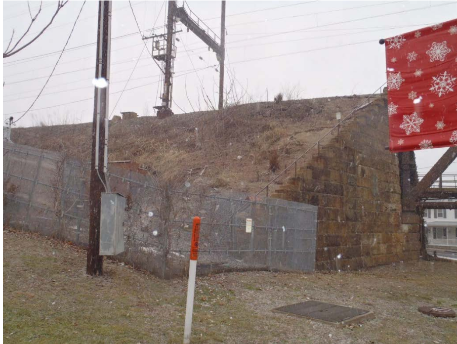
Photograph 3: General view of embankment supporting railroad and railroad bridge over St. John Street, facing southwest; Note the presence of multiple underground utilities within the vicinity of the berm.
