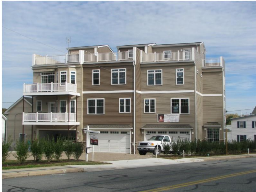
Photo 26: View looking northeast at a modern residential structure on Otsego Street.
