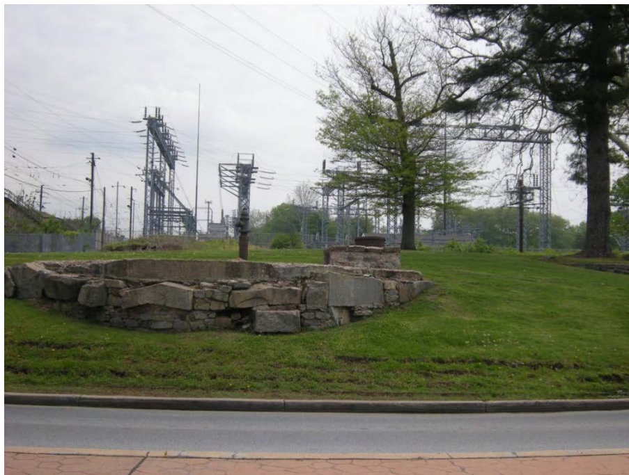
Photograph 31: View of southern portion of Study Area 4 with PW&B abutment, facing east.
