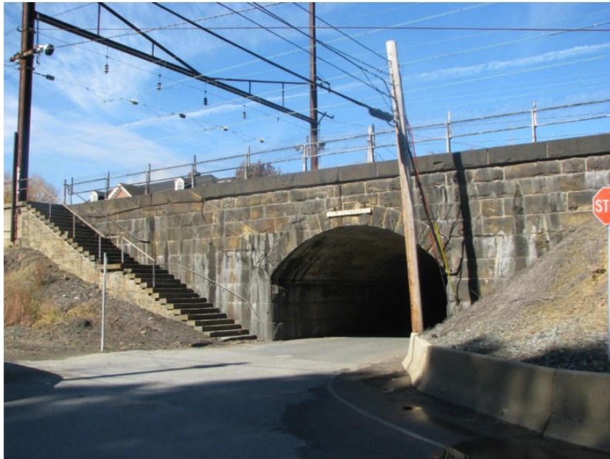
Photo 52: View looking at the east side of Perryville Railroad Station Undergrade Bridge (MP 59.39) that will be extended with a precast concrete culvert.
