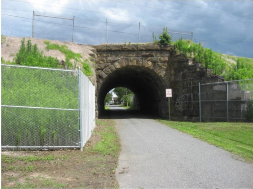
Photo 59: View looking north at the railroad east side of Centennial Lane Undergrade Bridge (MP 60.61), which will be extended with a precast concrete culvert and possibly altered via construction of a through plate girder bridge on a concrete abutment (for Alternate 9A only).
