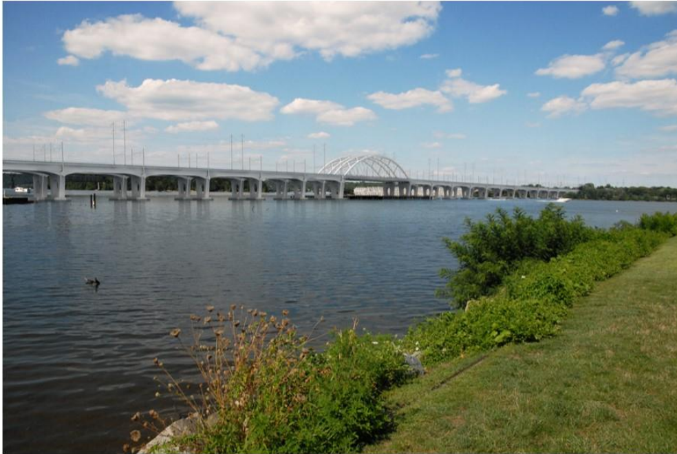
Photo 46: Rendering of a proposed replacement bridge with a girder approach and arch main span. View looking northeast from Havre de Grace.
