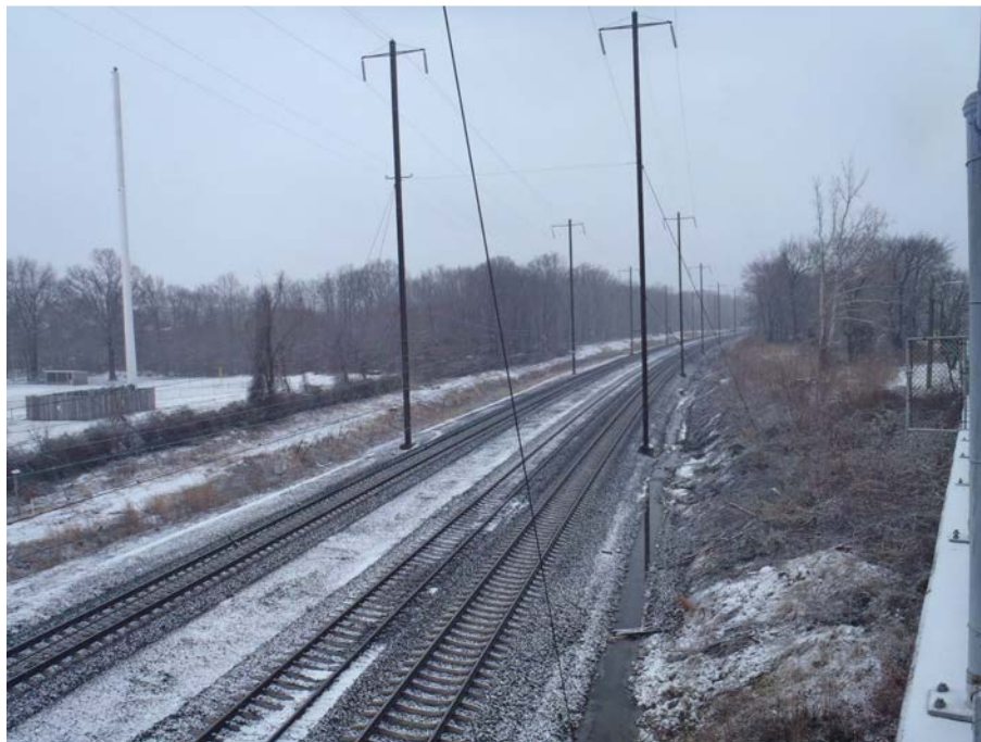
Photograph 8: General view of disturbed Amtrak ROW west of Revolution Street, facing west.
