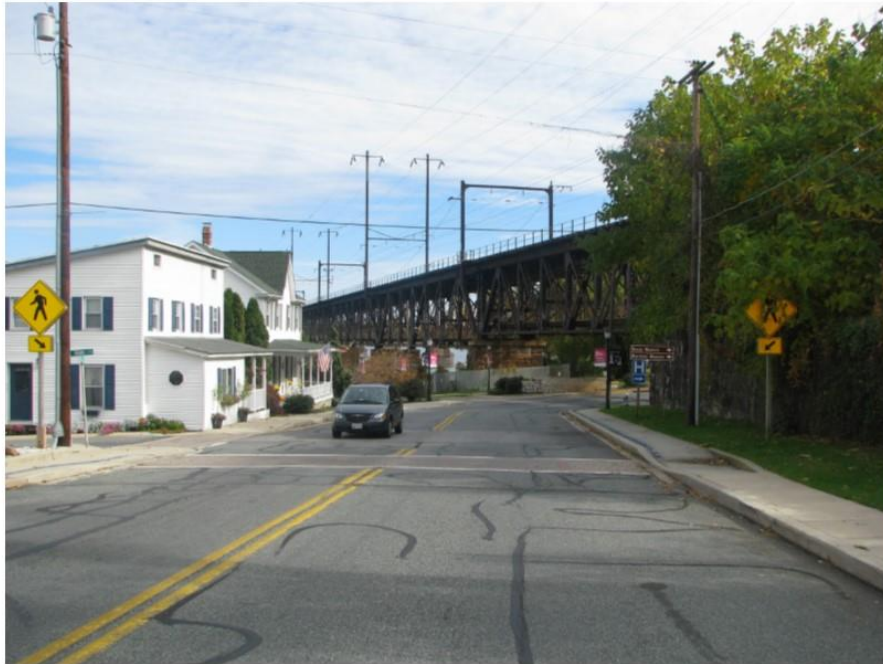
Photo 67: View looking east along Otsego Street at the houses located at the intersection of Otsego and Water Streets. The setting of these houses will be altered by the proposed widening that will bring the tracks 46-48 feet closer to them.
