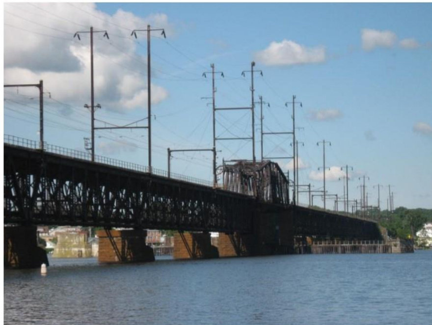
Photo 39: View looking northeast at the Susquehanna River Rail Bridge.
