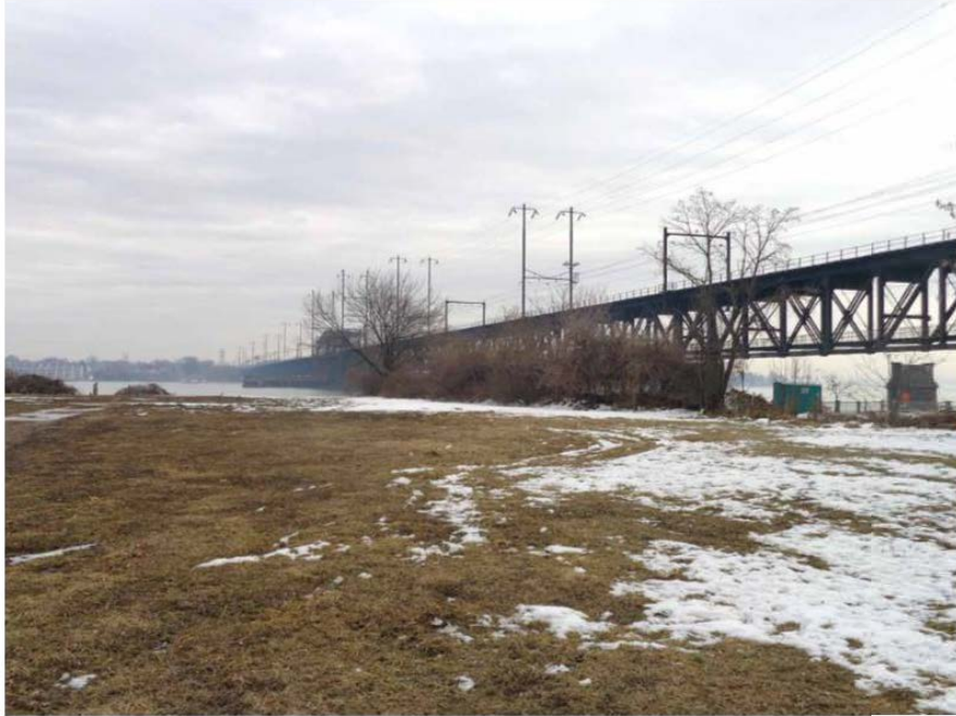
Photo 31: View looking east at the Jean S. Roberts Memorial Park along the waterfront immediately north of the Susquehanna River Rail Bridge.
