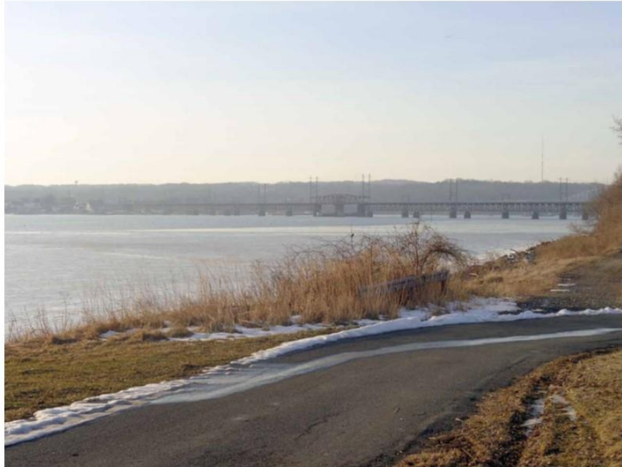
Photo 82: View looking northwest towards the Susquehanna River Rail Bridge from a waterfront walking path near the Perry Point Mansion and Mill.
