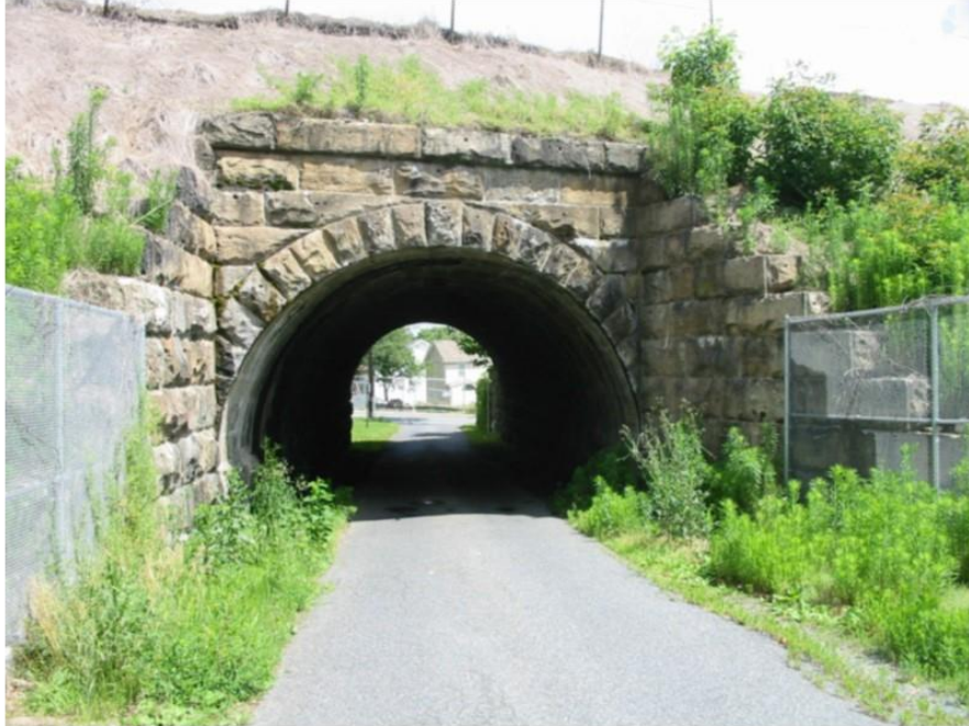
Photo 55: View looking north at the railroad east side of North Freedom Lane Undergrade Bridge (MP 60.51), which will be altered via construction of a precast concrete culvert.
