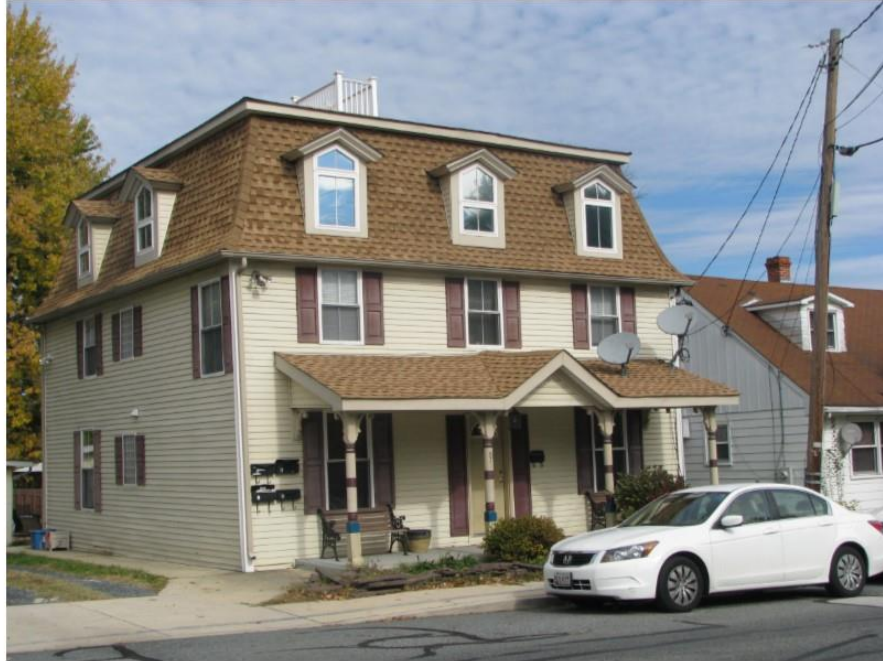
Photo 25: View looking north at an altered mid-nineteenth century French Second Empire house at 571 Otsego Street.
