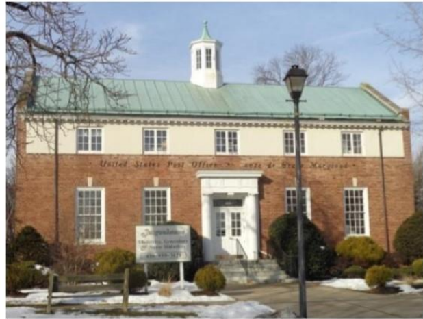
Photo 6: Representative masonry governmental structure within the Havre de Grace Historic District.
