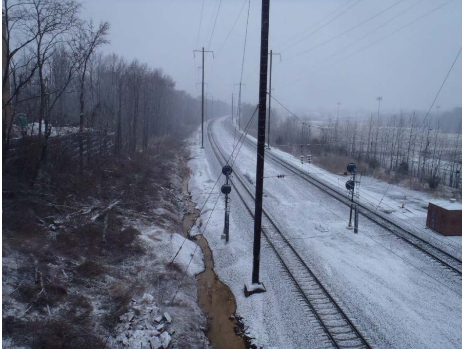
Photograph 5: General view of disturbed Amtrak ROW east of Lewis Lane, facing northeast.
