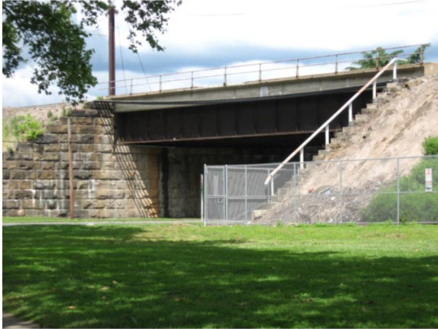
Photo 57: View looking northwest at the railroad east side of North Stokes Street Undergrade Bridge (MP 60.56), which will be altered via building a new concrete abutment.
