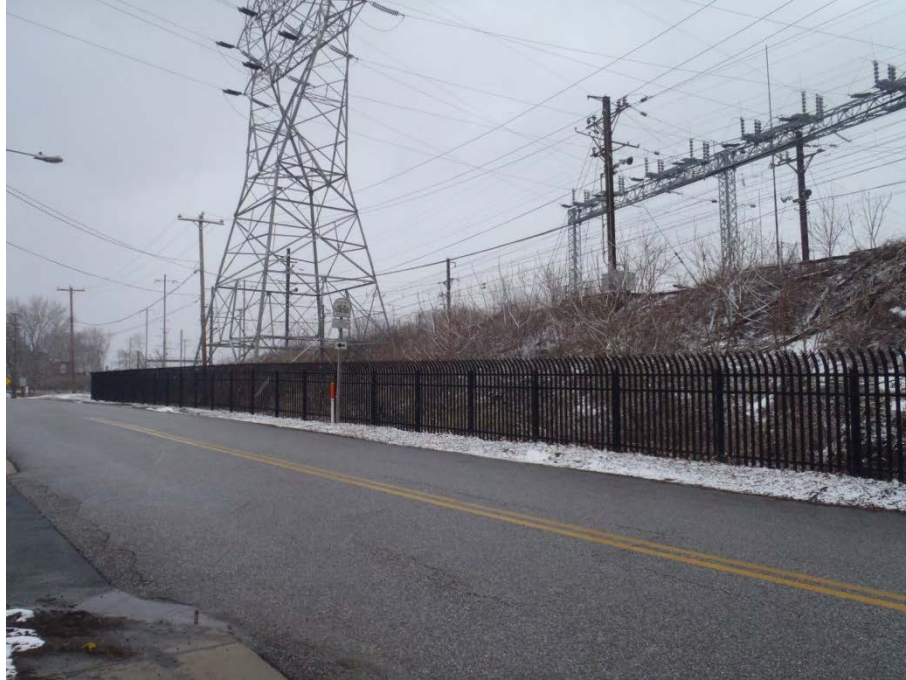
Photograph 9: General view of embankment south of Broad Street within Perryville, facing east.
