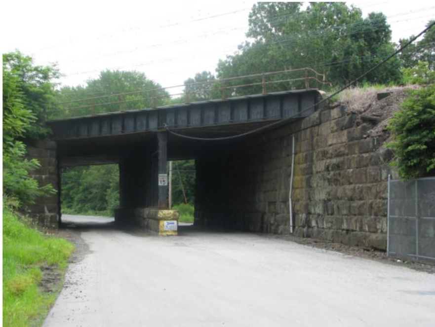
Photo 54: View looking southeast at the west side of the Access Road Undergrade Bridge (MP 59.52), which will be altered via replacing the existing structure with a precast concrete culvert (with a wider footprint) and partially demolishing and burying the abutments.
