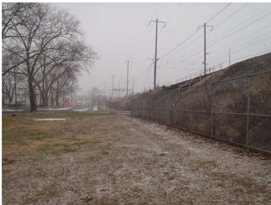
Photograph 4: General view of embankment supporting the elevated railroad corridor, facing southwest.
