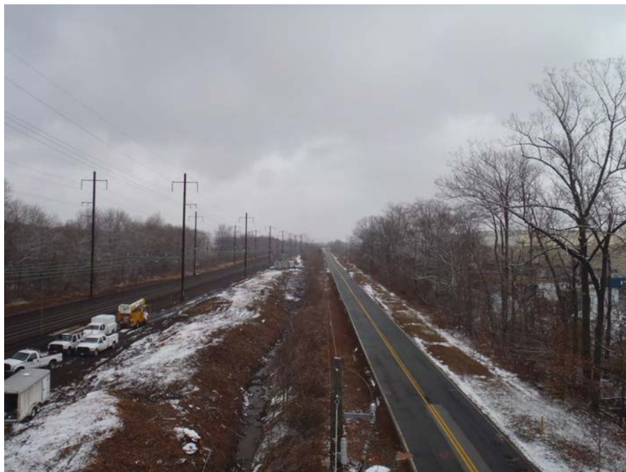
Photograph 12: General view of disturbed Amtrak ROW east of Firestone Road, facing east.
