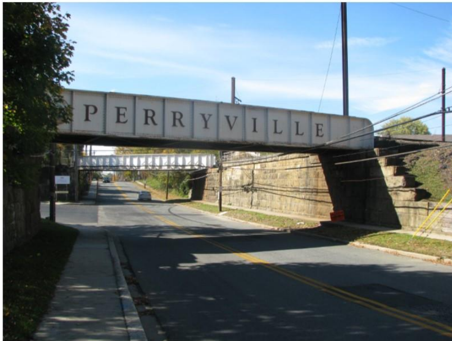
Photo 84: View looking west along Broad Street towards bridge carrying the south wye track over Broad Street.
