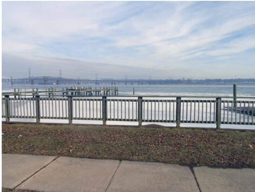
Photo 66: View looking northeast towards the Susquehanna River Rail Bridge from the Frank J. Hutchins Memorial Park, showing the bridge from one of the furthest points in the historic district within the APE.
