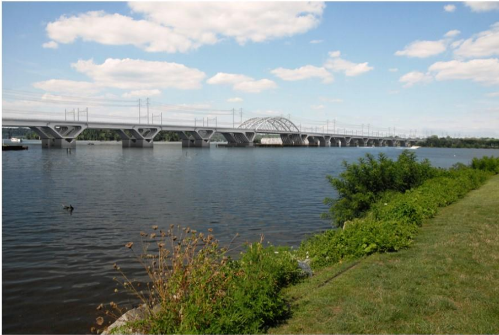
Photo 47: Rendering of a proposed replacement bridge with a Delta frame approach and arch main span. View looking northeast from Havre de Grace.
