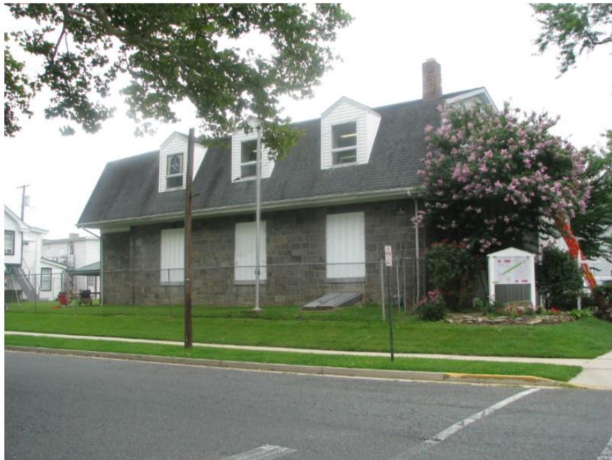
Photo 14: View looking southeast at the Room at the Cross Mission Church, the former St. Patrick's Catholic Church, 429 N. Stokes Street.
